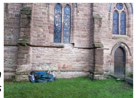
String course work in progress
